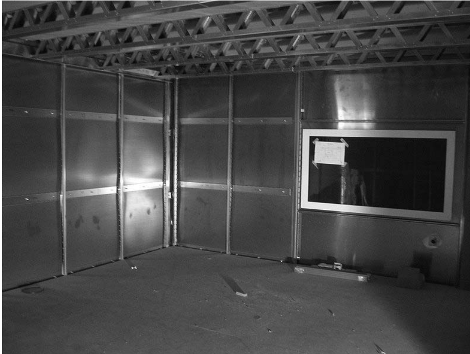
Figure 17: An example Faraday cage. (Image by M. Junghans; licenced under the terms of the GNU Free Documentation License, Version 1.2.)
